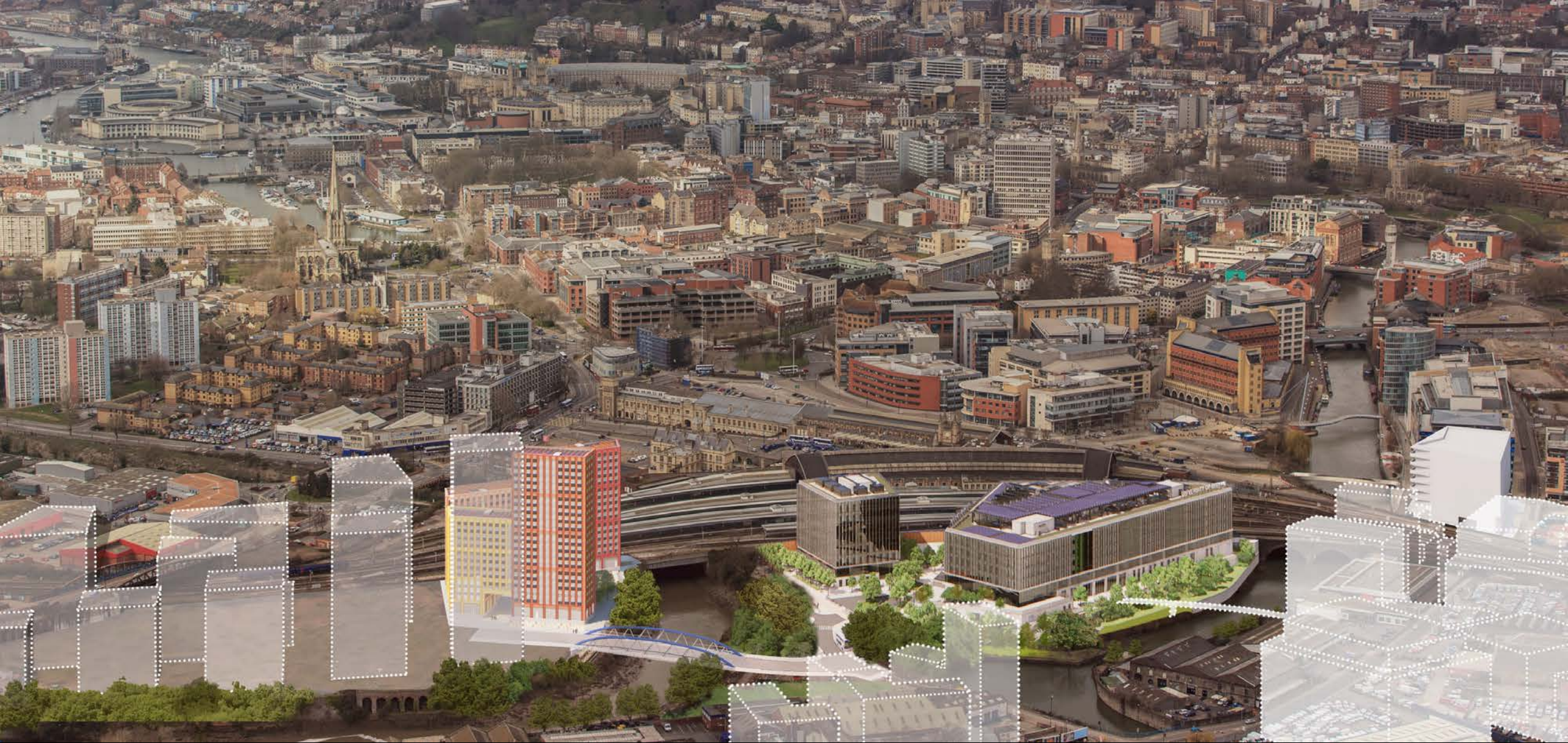
Aerial view of the Temple Quarter Enterprise Campus
